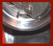
Brush Plating repair done during an outage in 3hours of work at the reactor face.
