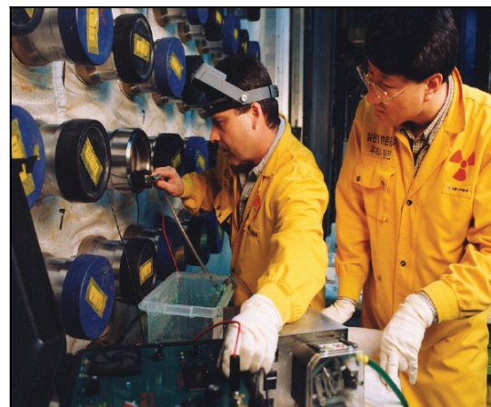
Repair of E-Face surface prior to the start up at Wolsong 2, South Korea (2002).
