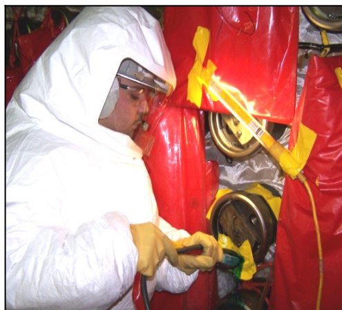
In-situ repair performed on End Fitting at Bruce Nuclear Power, Ontario (2005).
